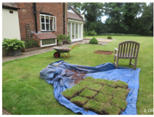
Step 1: Remove any turf and put it to one side.
